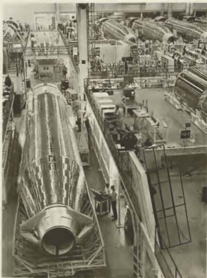
The two major systems of Mercury flight hardware were of course the launch vehicle—the man-rated Atlas—being produced at General Dynamics/Astronautics plant in San Diego (left) and the Mercury spacecraft, being assembled at the McDonnell Aircraft Corporation plant in St. Louis (below).
