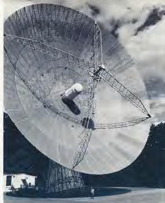
**Paul Horowitz' six-year-old son, Jacob, reaches up toward the 84-foot dish of the radio telescope at Harvard's Oak Ridge Observatory. This facility has been refurbished and sensitive signal acquisition equipment assembled with funds provided by The Planetary Society. The Planetary Society/Harvard SETI program is the most comprehensive and sensitive such effort ever attempted.**
