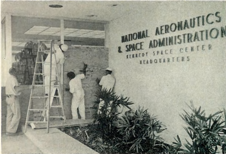
TWA WORKMEN boarded up large plate glass in front of the KSC Headquarters Building when Hurricane Betsy looked like it might sideswipe the area. In other areas throughout the Center windows were boarded and low ground areas were sandbagged.
