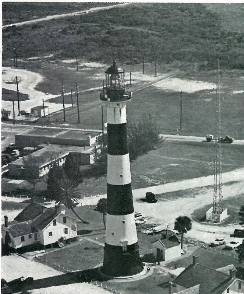
SURROUNDED by gantrys and other signs of the space age, the 165-foot lighthouse dates back to 1868. First light was a kerosene lamp, magnified by prisms.
