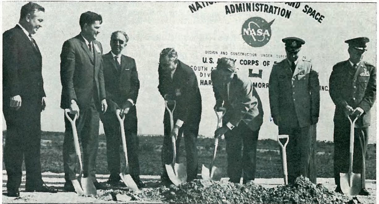
DIGGING IN at ground-breaking ceremonies Monday for the new Manned Spacecraft Operations and Checkout Building on Merritt Island were these NASA and military officials. Left to right are Walter C. Williams, MSC Associate Director; G. Merritt Preston, Director of MSC Pre-flight Operations; Dr. Kurt Debus, LOC Director; D. Brainerd Holmes, Director, Office of Manned Spaceflight; Dr. Wernher von Braun, Director, Marshall Space Flight Center; Col. H. R. Parfitt, U. S. Army District Engineer; and Col. E. Richardson, Air Force Missile Test Center representative.
