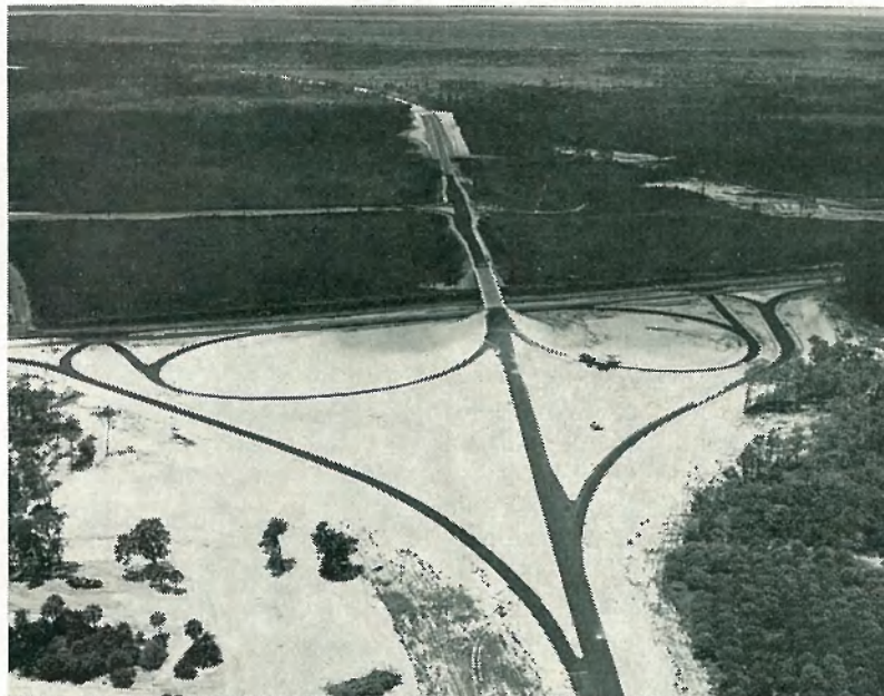
CAPE CANAVERAL Causeway cloverleaf at U.S. 1 intersection shows how north and south bound traffic will feed into main flow. The Causeway is expected to open next month.
