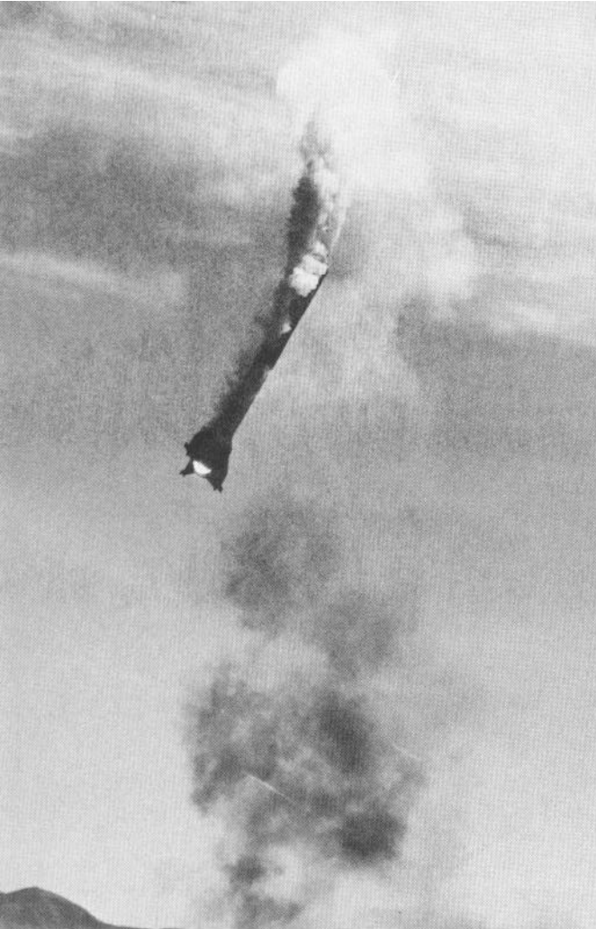
On opposite page, a V-1 explodes during 1948 attempt to launch the missile from a submarine, the USS Cusk (SS-348). These experiments paved the way for the Regulus program.
