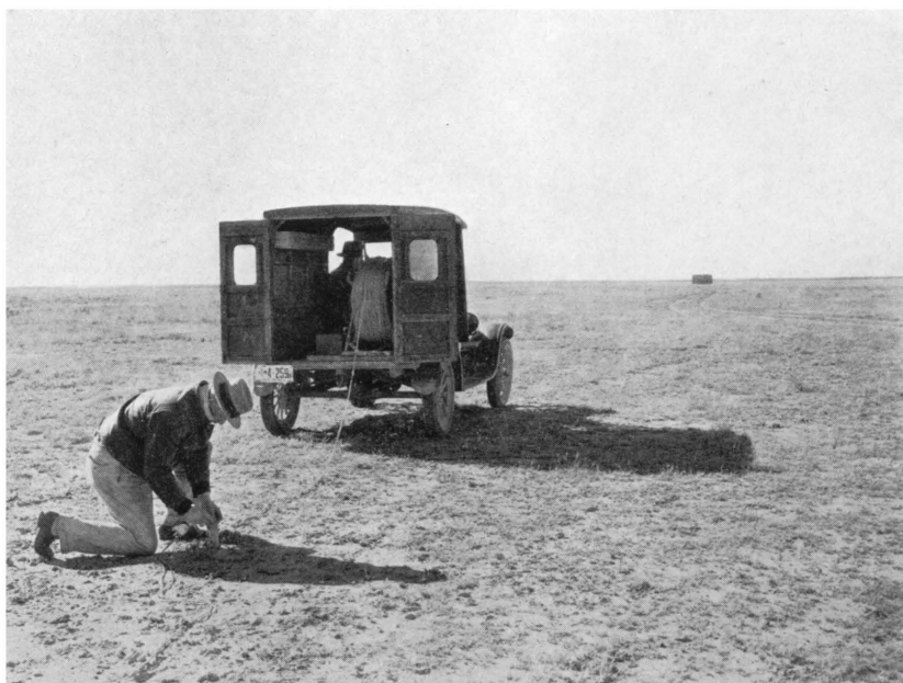
2. Cable being unspooled between the tower and the 1,000-foot shelter.
