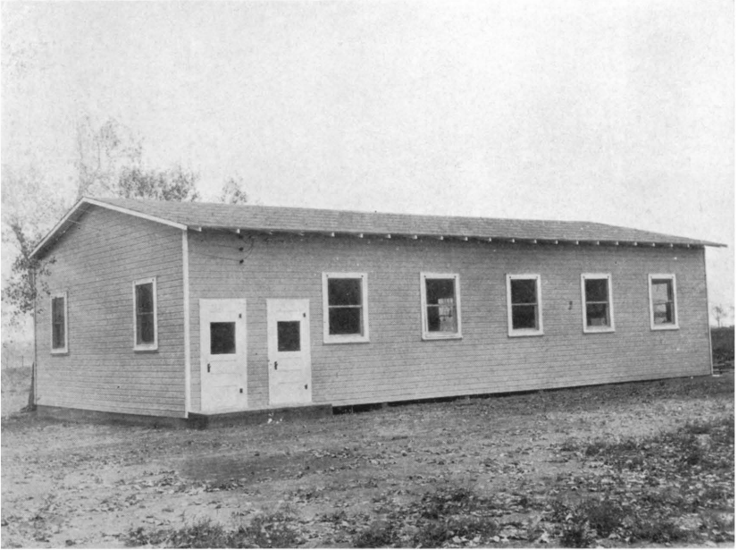
1. Shop erected at Roswell, N. Mex., in September 1930.
