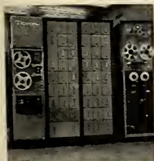
DEMON Automatic checkout system built by Curtiss-Wright is used on Nike-Ajax (see p. 33).
