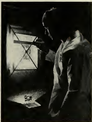
ORIGINAL artwork for printed circuits in sub-miniature assemblies is drawn twice desired size, reduced photographically. Ryan technician checks camera.
