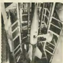
BRITAIN's Thunderbird undergoes six foot drop test to simulate shock of launching at English Electric's facility.
