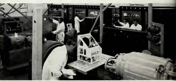
Typical installation of Ling Vibration Testing System installed i Missile Development Division of North American Aviation.
