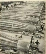
FIRST production line photograph of Atlas ICBM at Convair shows vehicles to be fired in the test program and similar missiles for operational use.
