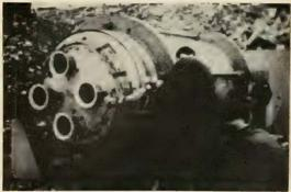
JETEVATORS ON EACH of the four nozzles in AX Polaris series are formed from two gimballed rings to deflect thrust.
