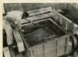
SOLIDS mixer by Baker Perkins is boosting propellant output for Thiokol Chemical Co. (p. 26)
