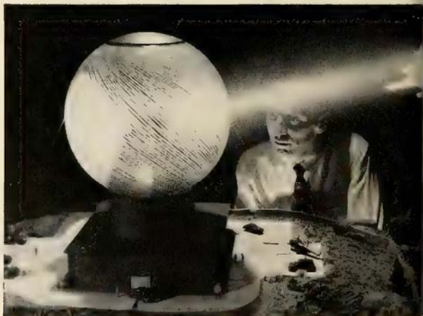
NON-ROTATING 360° RADAR ANTENNA. Only the feed point moves. Principle involved will permit economical construction of very large high gain scanning antennas. Application of inflation techniques will permit lighter-weight long-range air-transportable radar. Working models already built and evaluated. Electronic Division and Research Laboratories
