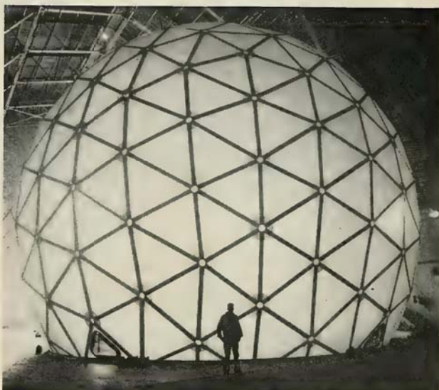
"WORLD'S LARGEST" fiberglass radome designed and built by Goodyear Aircraft Corp. for the Missile Detection Systems Section of GE, measures 68 feet in diameter and stands more than seven stories high. It can be erected by six men in 80 hours.
