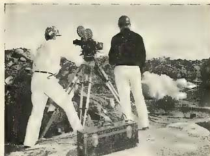
Precision Test Firing of Rocket Engine at Rocketdyne's Propulsion Field Laboratory is recorded by Mitchell Camera in remote 1600 acre test area in Santa Susana Mountains, California.
