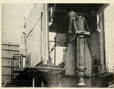
THIS 19 FOOT liquid powerplant has been installed at Reaction Motors' Lake Denmark, N.J. for test and evaluation. As an example of the short development time involved in building packaged powerplants in different sizes, this large unit was first tested within three months of the time work was begun on the Guardian engine project.
