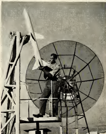
ANTENNA SYSTEM on missile model being checked at Electronic Specialty Co.'s test facility.
