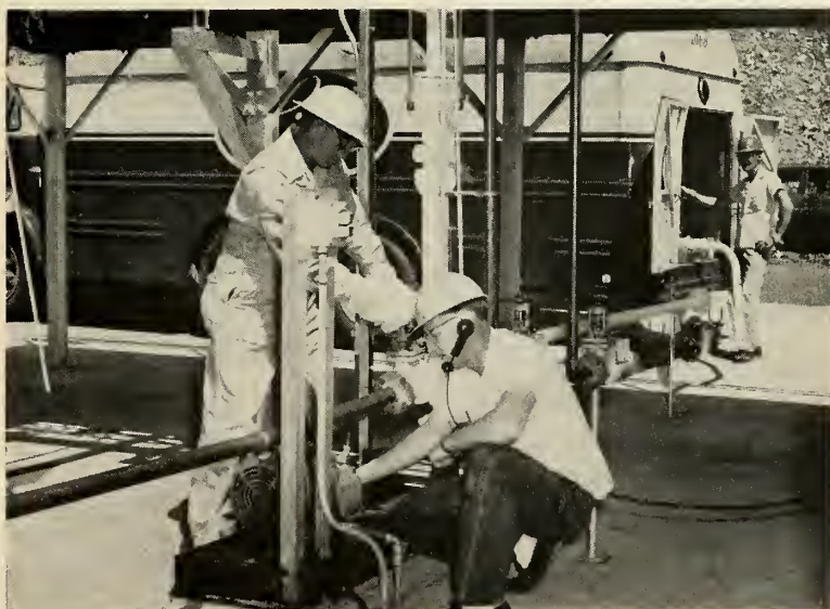
TECHNICIANS TRANSFER LOX with pumps from truck to storage tanks at Rocket-dyne's Neosho plant.
