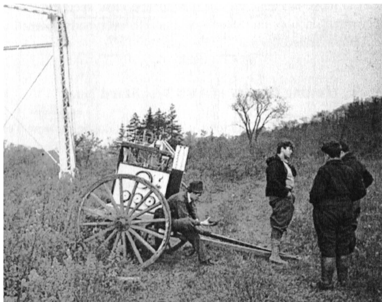
Figure 15–6: Another rare photo, taken by James Wyld in 1938, showing a specially-built cart for hauling ARS Test Stand No. 2 to its chosen test sites. The Stand was “portable” but still weighed some 300 lb (136 kg). Taken 21 October 1938 near the test site at New Rochelle, New York. Credit: Smithsonian photo 9A05175.
