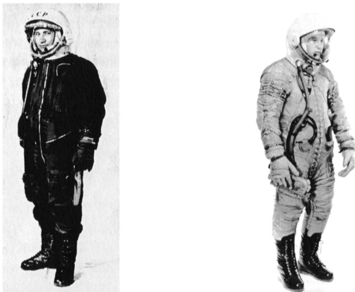
Figures 8a and 8b: Left, SK-1 full pressure suit used by Yuri A. Gagarin. Here with test person Yuri Orekhov; Right, SK-1 space-suit without the protective overall. Here with test person Victor Yefimov ( Archive Zvezda ).
