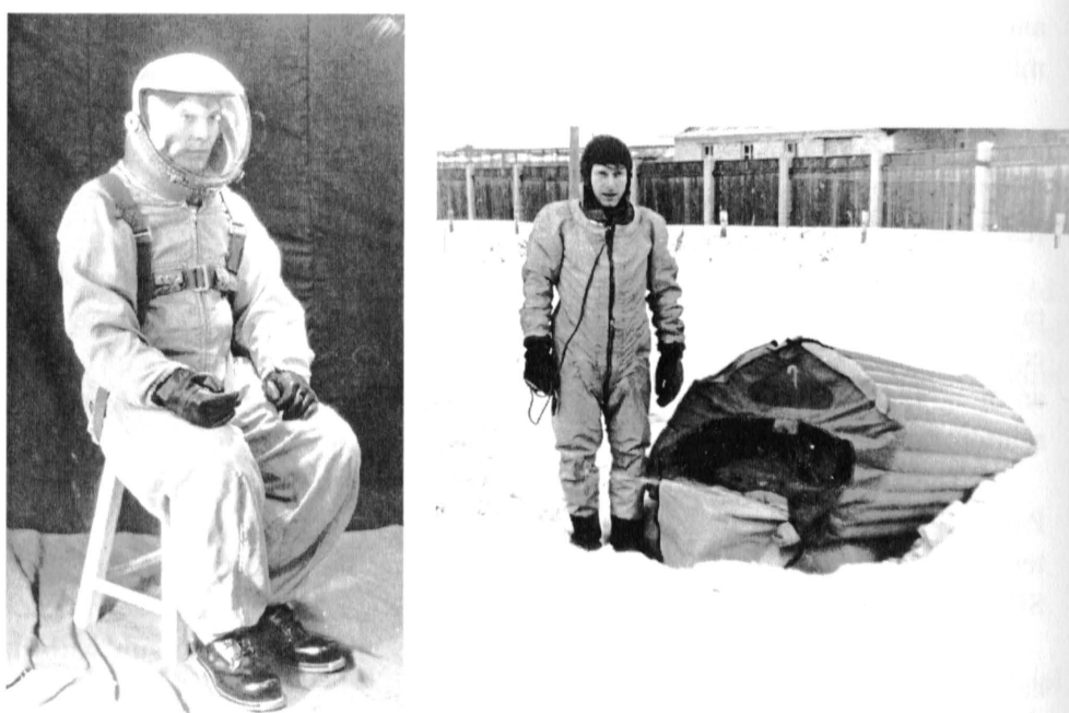
Figures 5 and 6: Left, general view of S-10 space-suit breadboard in 1959. Right, Testing of the V-3 protective suit under winter conditions ( Archive Zvezda ).
