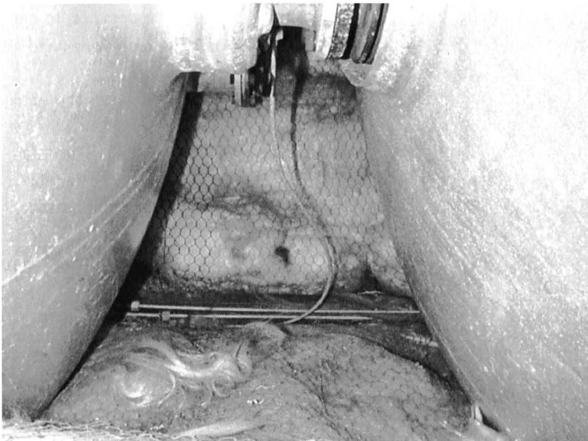
Figure 8: Glass wool insulation was packed around the fuel and oxidant tanks and held in with chicken wire.
