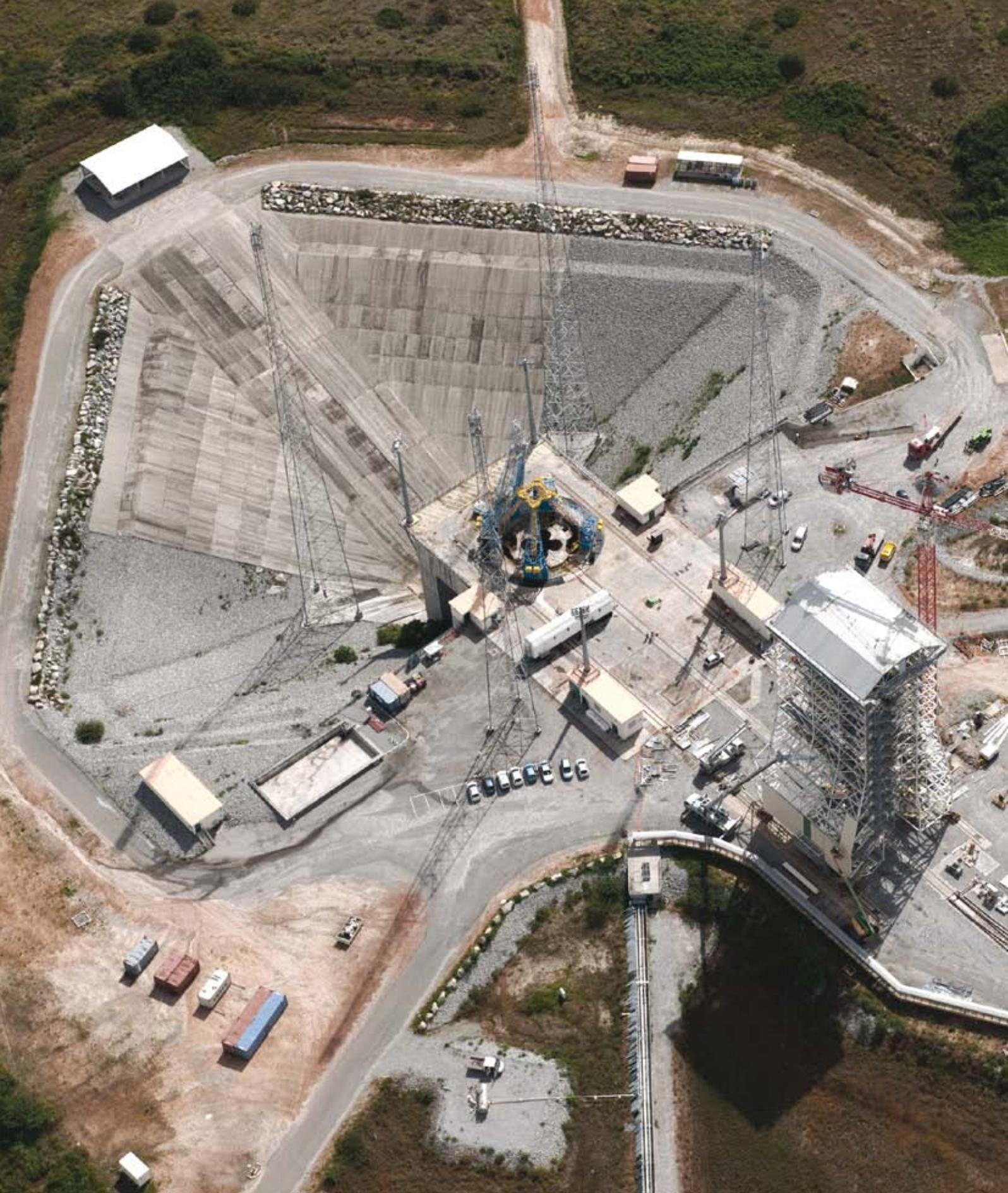
The new Soyuz launch facility at the Centre Spatial Guyana (CSG), Europe's Spaceport in French Guiana, with a view of the Soyuz launch platform from the flame pit. This five-level reinforced concrete structure houses mission equipment. The top two levels have 15 m-wide openings for the launch table and the erected Soyuz vehicle. Its upper area accommodates the pad infrastructure, including the service tower, the fuelling booms and the erector (ESA/CNES/Arianespace/Optique Video CSG)
