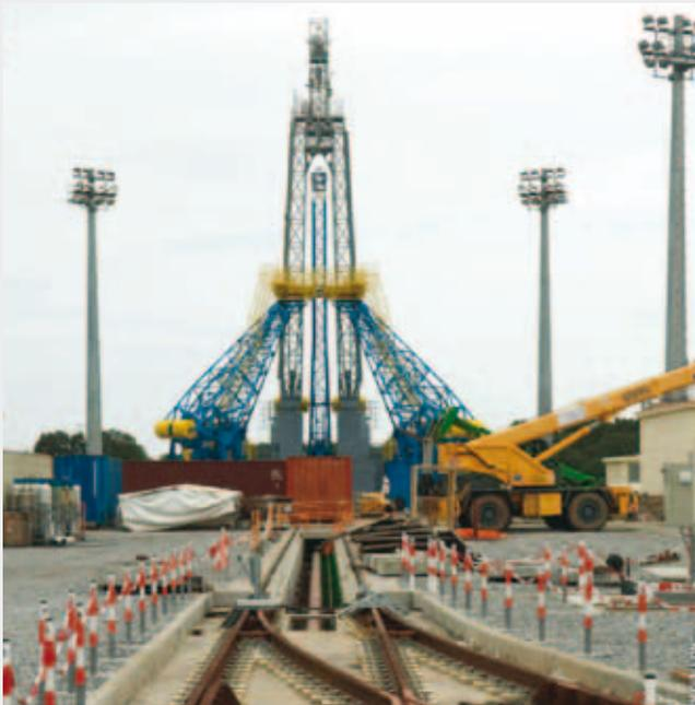
The new Soyuz launch pad in the 'ready' position, i.e. with the four support arms closed and the two umbilical masts raised to service the Soyuz vehicle, viewed from the railtrack that will be used for the rollout of launch vehicles on their transporter/erector wagons (ESA/CNES/Arianespace/Optique vidéo du CSG/J. Guillon)
