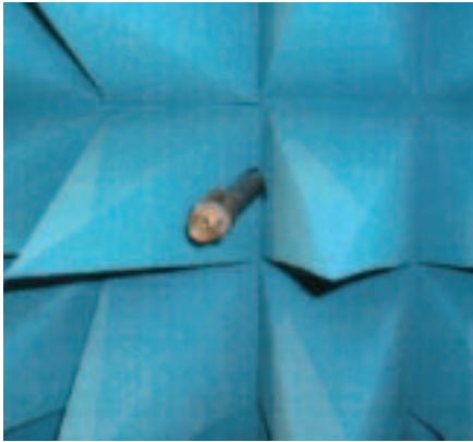
One of the many fire-extinguisher nozzles in the new chamber
