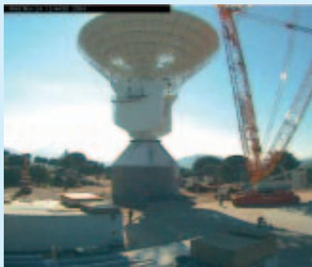
*Mounting of the antenna dish at ESA's Cebreros deep-space ground station in Spain*
