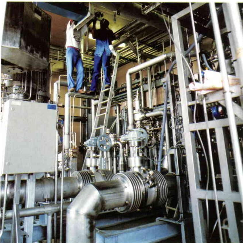
**Figure 12.** Inside the low terminal building, with the cryogenic feeding lines and all electrical and control systems for an automated, remote countdown management from the Control Centre (Photo: Bernard Paris)
