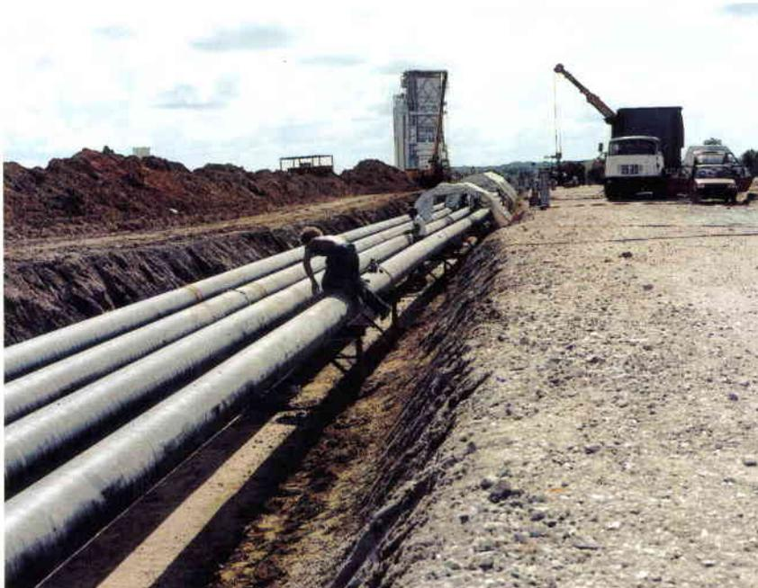
**Figure 3. The underground helium storage network being built (Photo: Bernard Paris)**
