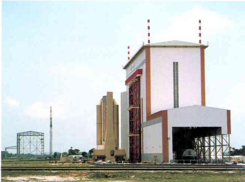
**Figure 5. The Launcher Integration Building (BIL) with the storage hall in the foreground. A mockup of the lower composite has been rolled out of the integration hall on a mobile launch platform. In the background, the Final Assembly Building is under construction (September 1993) (Photo: Bernard Paris)**
