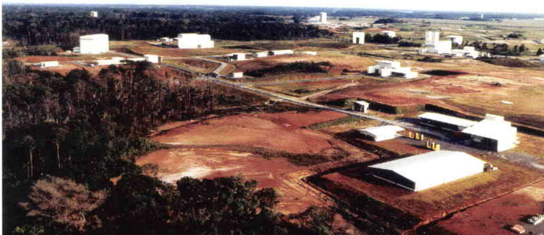
Figure 5. View of part of the UPG, with the Booster Integration Building and the top of the Test Stand in the background
