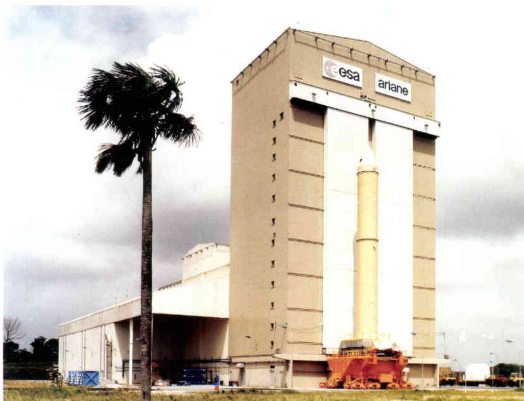
Figure 6. The Booster Integration Building (BIP)
