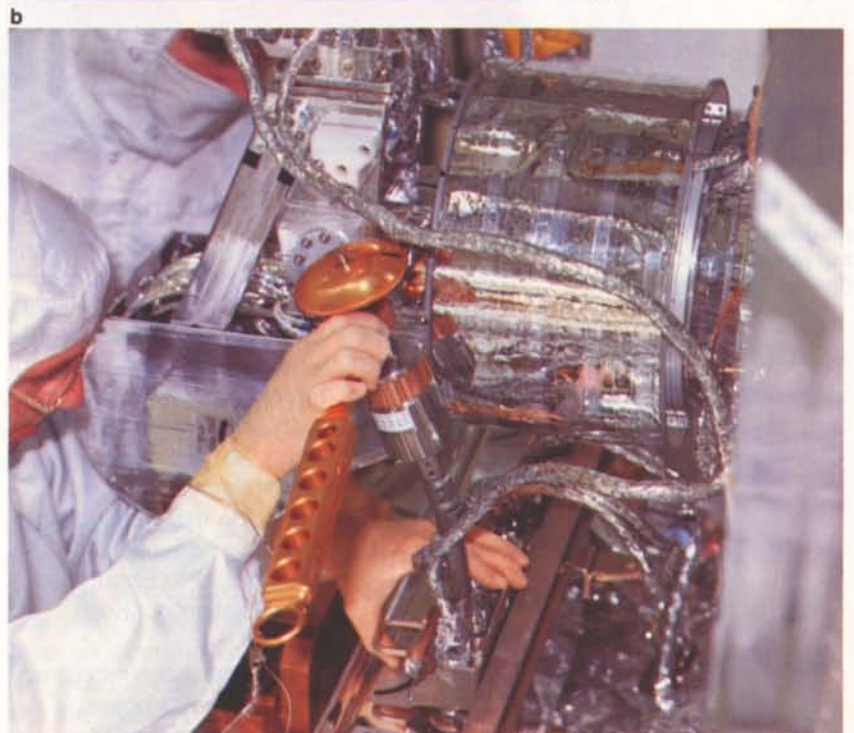
Figure 6. Fitting of Diode Box Connectors with a manual tool and torque limiter, illustrating the benefit of the 'wobble drive'
