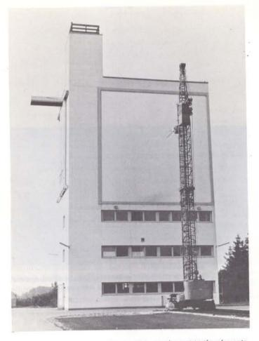
Figure 6 – To avoid exposing antennas under test to the elements, one wall of MBB's anechoic chamber (top of building) is transparent to radio frequencies. The movable tower allows testing at various distances.
