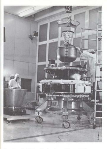
Figure 3 – Installation of inert motor model in spacecraft.
