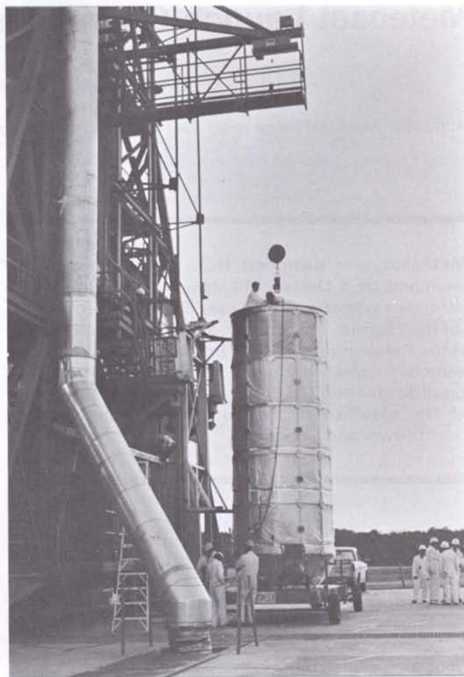
Figure 4 – Hoisting the 'yellow can' – containing the satellite, ABM and third stage – up the side of the gantry.
