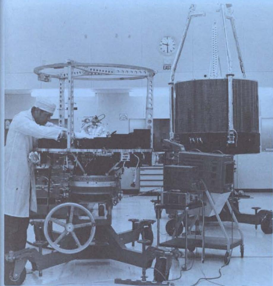
ISEE-B flight model in clean room at ESTEC.
