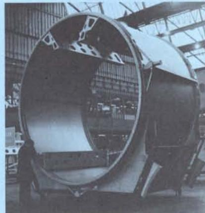
*Spacelab cylindrical module, at Aeritalia, showing storage and floor attachments.*
