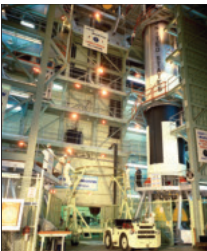
In 1966, Martin Baltimore technicians hoist the second stage of the Gemini IX Titan II into position for test. A dozen of the Air Force ICBMs were modified for Gemini launch duties; the Middle River-assembled Titans had a perfect flight record. Courtesy GLMMAM.
