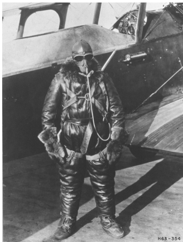
Figure 2.2. 1920s' NACA/U.S. Army Air Corp oxygen mask and thermal protection suit (courtesy Hamilton Sundstrand).
