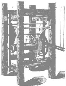
the arm B out of its notch in the locking plate C. The stop D, called, I believe, the nag's head, being on the same spindle as B, is at the same time raised, and mounts on to a plate going partly round the edges of the wheel F. The fly E, after making nearly a turn, is checked by a pin in the lever A, and the train can not go on until the lever A, is freed from the going part of the clock at the quarter. The inner end of the lever A then
