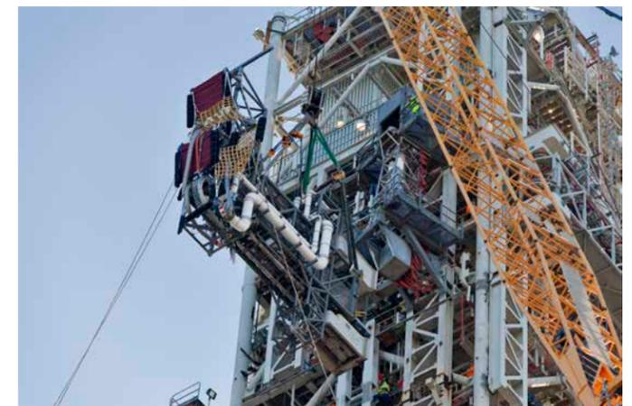
A heavy-lift crane and rigging lines are used to lift the Interim Cryogenic Propulsion Stage Umbilical high up for installation on the tower of the mobile launcher on March 16, 2018, at NASA's Kennedy Space Center. Photo credit: NASA/Ben Smegelsky
