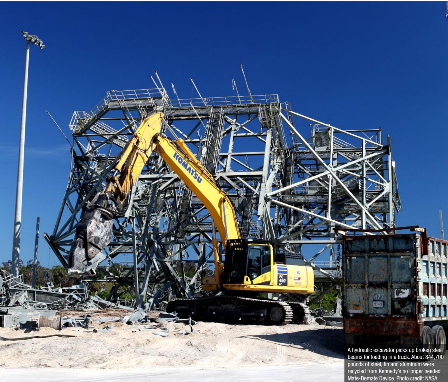
A hydraulic excavator picks up broken steel beams for loading in a truck. About 844,700 pounds of steel, tin and aluminum were recycled from Kennedy’s no longer needed Mate-Demate Device. Photo credit: NASA
