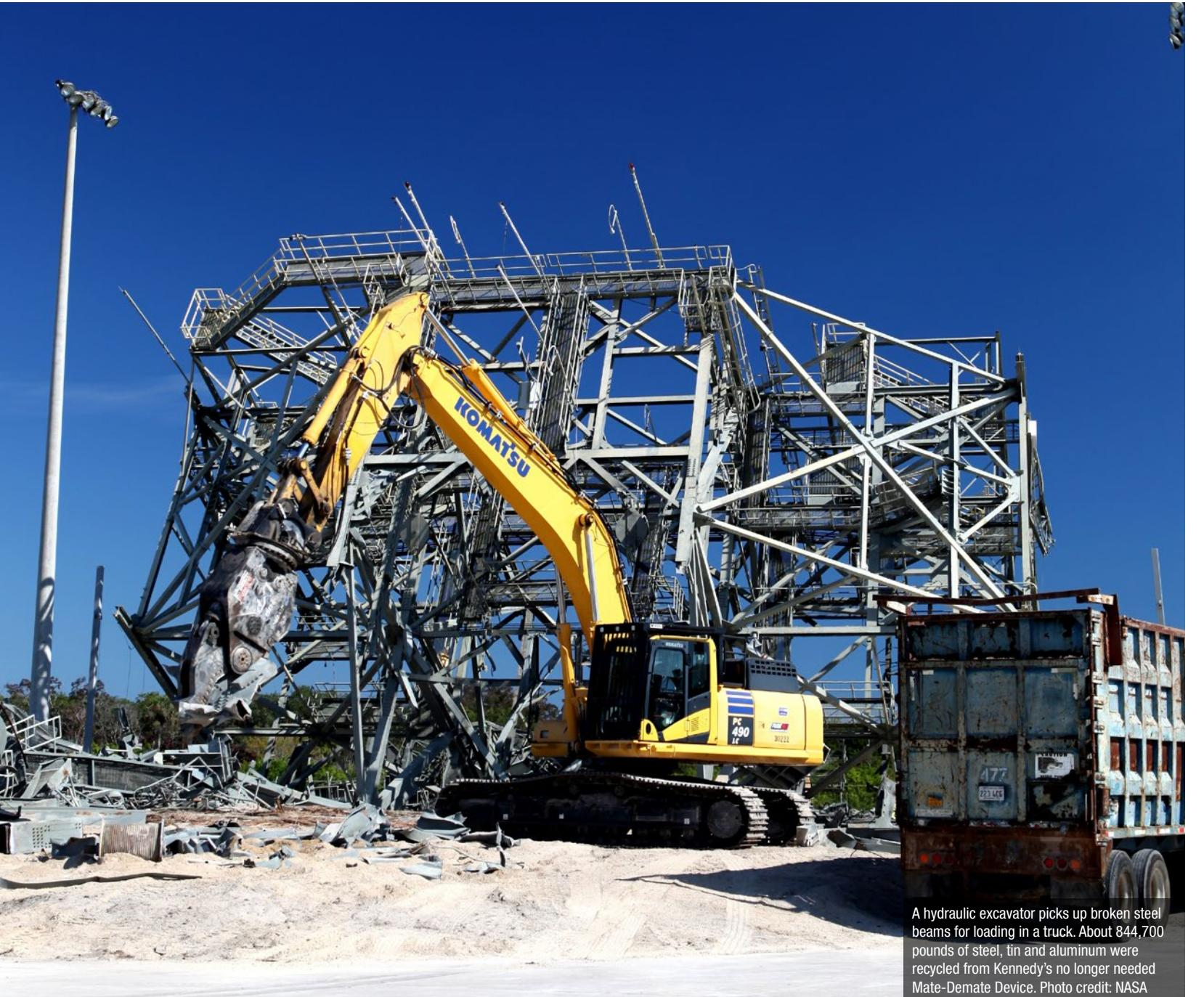
A hydraulic excavator picks up broken steel beams for loading in a truck. About 844,700 pounds of steel, tin and aluminum were recycled from Kennedy's no longer needed Mate-Demate Device. Photo credit: NASA
