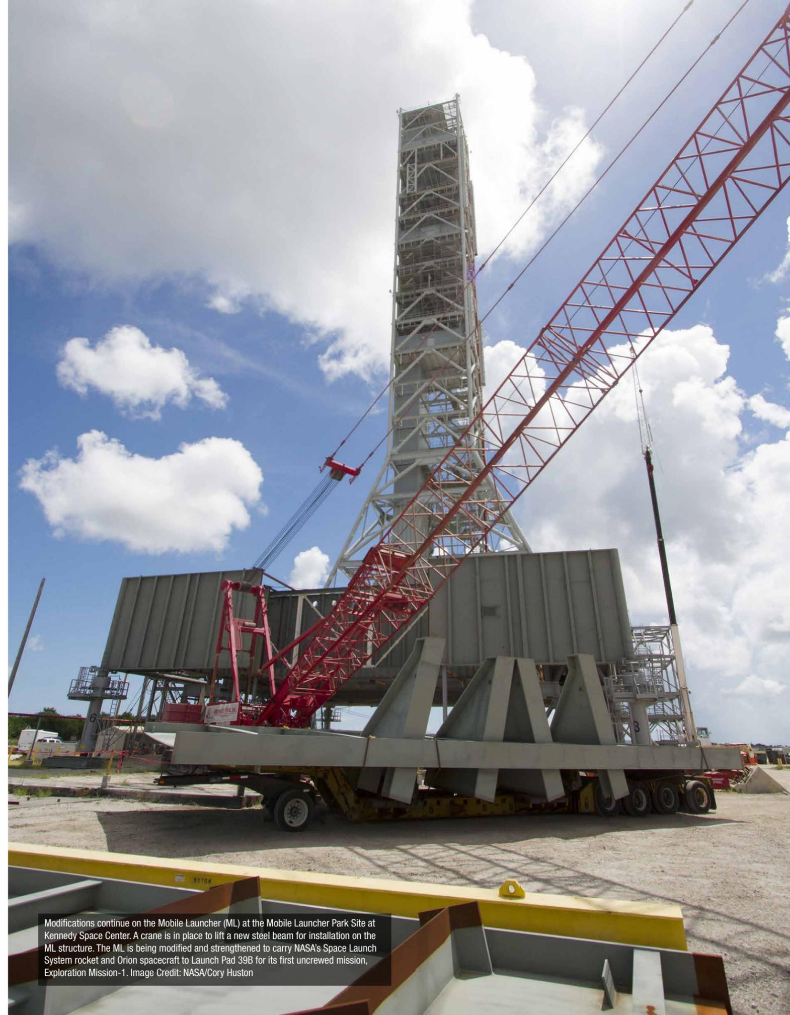
Modifications continue on the Mobile Launcher (ML) at the Mobile Launcher Park Site at Kennedy Space Center. A crane is in place to lift a new steel beam for installation on the ML structure. The ML is being modified and strengthened to carry NASA's Space Launch System rocket and Orion spacecraft to Launch Pad 39B for its first uncrewed mission, Exploration Mission-1. Image Credit: NASA/Cory Huston
