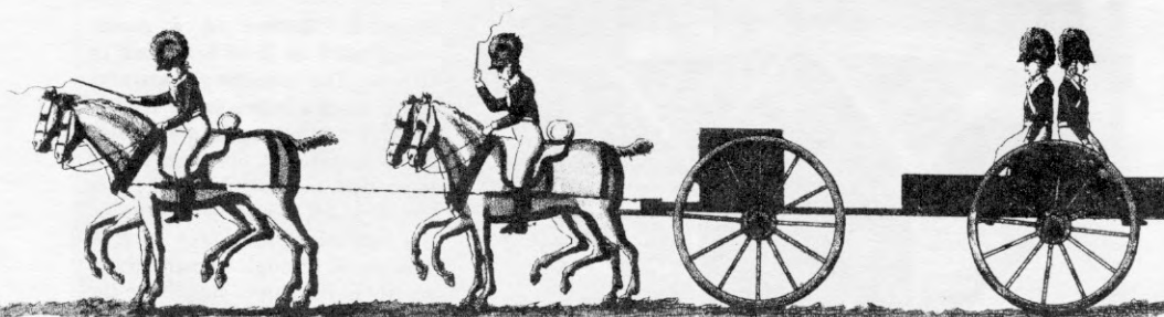
Figure 9. This specially designed "rocket car" was constructed in two sections — one to carry the warheads and projectiles, the other to carry the launching sticks. Equipment like this was used by R.H.A. rocket troops in Spain and North America in 1813-1815 who were equipped with the medium caliber rockets.
