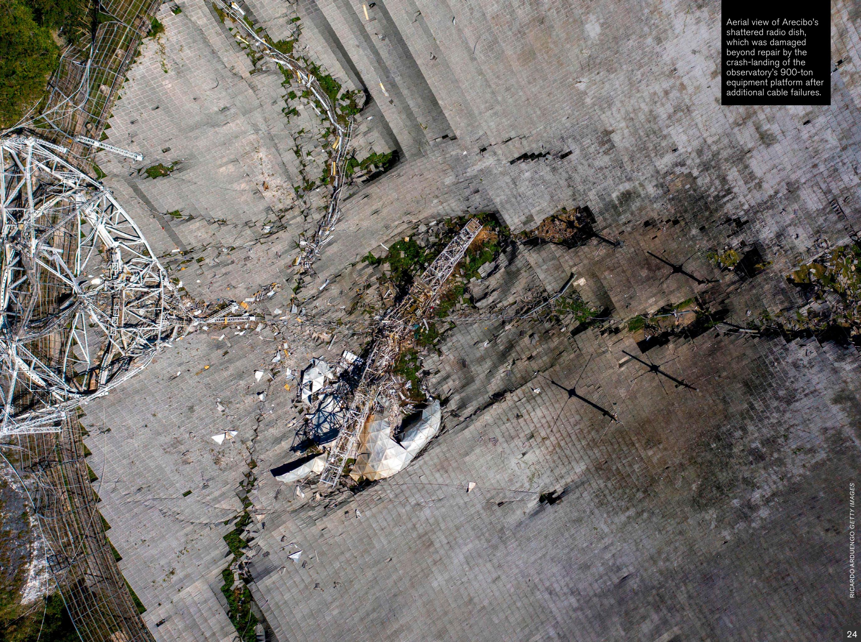
Aerial view of Arecibo's shattered radio dish, which was damaged beyond repair by the crash-landing of the observatory's 900-ton equipment platform after additional cable failures.
