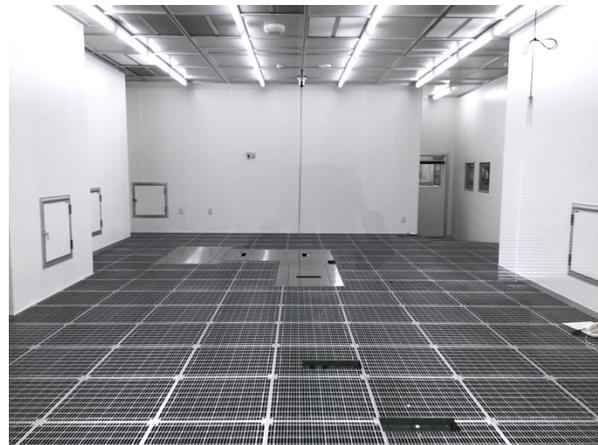
Fig. 2. A newly renovated clean room for O-REX returned samples. Its cleanliness level is ISO 6. It has a grating floor and a base for new CCs, which is under development and will be installed there in fall 2023.
