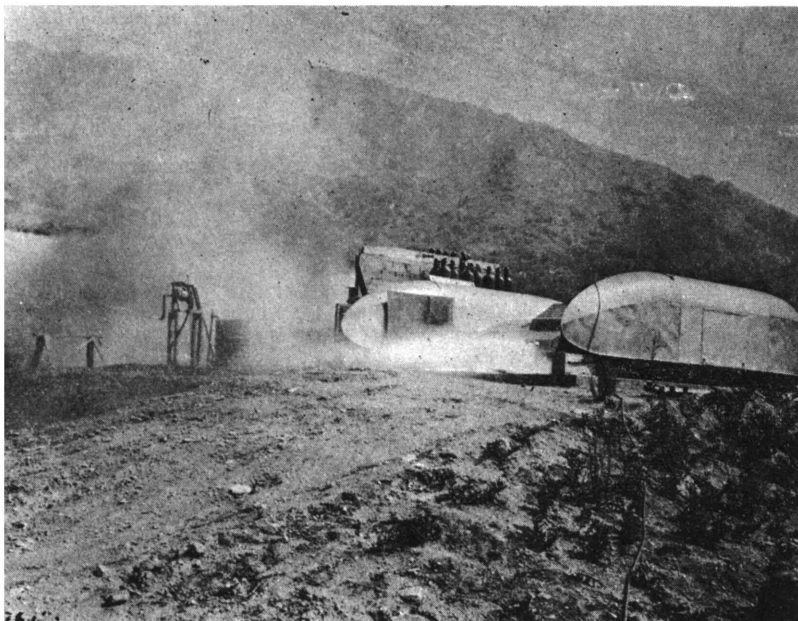
Static test of rocket propelled towing car.
