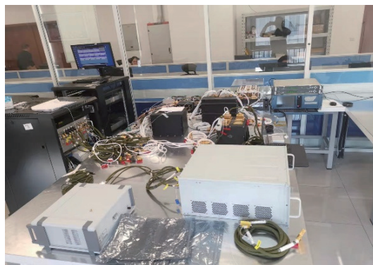
Fig. 10 PF electrical interface test
