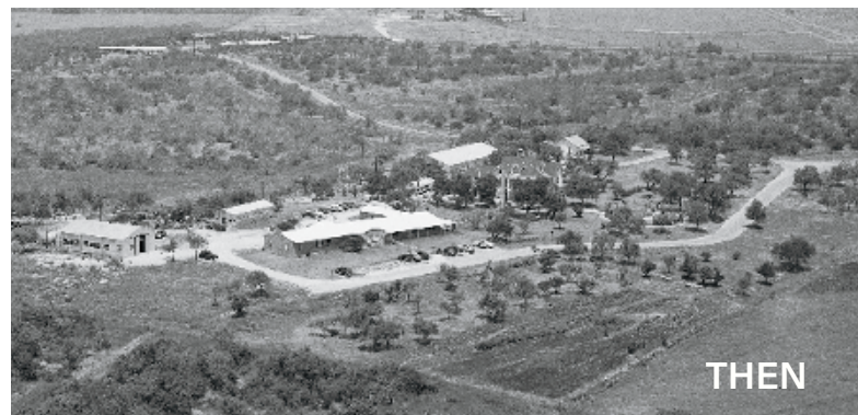
In 1947, SwRI was founded on the grounds of the Essar Ranch west of San Antonio, in six buildings with a total of 23,500 square feet (2,183 square meters). SWRI
