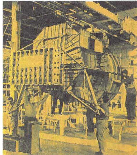
**Figure 22–34 (right):** LM Ascent Stage (rear) welding [Sciaky at Work Vol. 9 no. 2].
