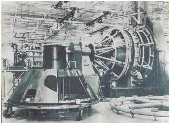
**Figure 22–31 (left):** CM positioner [Sciaky at Work Vol. 8 no. 10].
