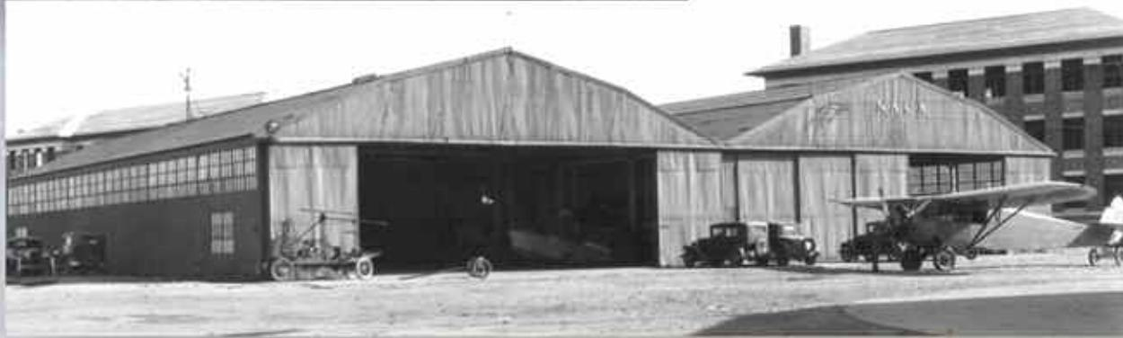
*Above: These are the original NACA aircraft hangars, photographed at Langley Research Center in 1931. The plane parked to the right is the Fairchild owned by NACA. Just outside the hangar door is a modified Ford Model A that was used to start aircraft engines.*
