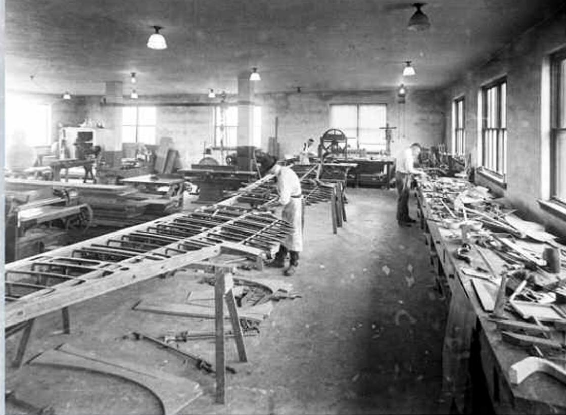
*Workmen in the Langley Research Center's pattern makers' shop manufacture a wing skeleton for a Thomas-Morse MB-3 airplane in June 1922. The airplane was used for pressure distribution studies in flight.*
