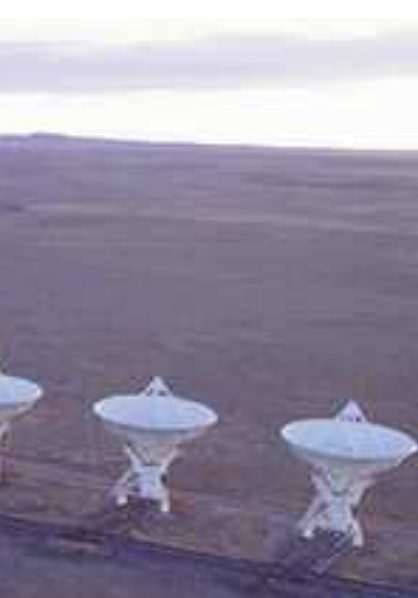
Twilight settles on the Very Large Array—27 radio antennae, each one measuring 25 meters in diameter, that form a giant Y-shape complex in the New Mexico plains. The data from the antennae are combined electronically to give the resolution of an antenna 36 kilometers (22 miles) across with the sensitivity of a dish 130 meters in diameter.
