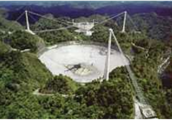
The Arecibo Observatory in Puerto Rico operates the world's largest, most sensitive radio telescope. This gigantic instrument consists of a large collecting surface, the suspended receiving elements, and an array of signal-processing equipment. Unlike most telescopes, which point by shifting the main mirror or reflector, the Arecibo telescope tracks celestial objects by moving the receiving elements suspended above the stationary reflector.
