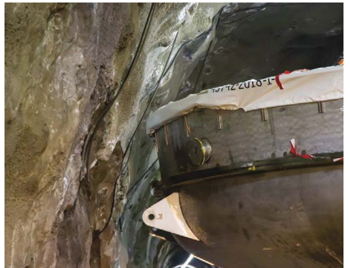
▲ TIGHT SQUEEZE After arriving at the port of Coquimbo in Chile in 2018, the telescope’s coating chamber was divided into two parts like an Oreo and transported to the summit of Cerro Pachón. Along the way, hanging signs, utility cables, and lights had to be removed to make room. Here, the chamber makes its way through the narrowest tunnel along the route. (Planners decided the telescope’s size with this tunnel in mind.)
