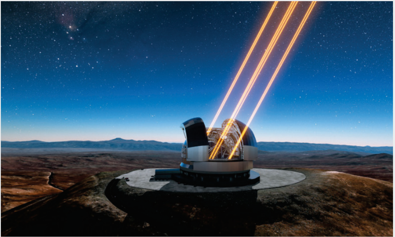
This artist's rendering shows the Extremely Large Telescope in operation on Cerro Armazones in northern Chile. The telescope will use lasers to create artificial stars high in the atmosphere.
