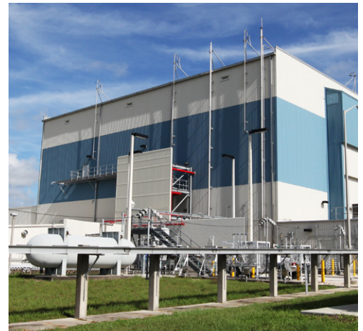
8 MULTI-PAYLOAD PROCESSING FACILITY PROVIDES 'GAS STATION' FOR ORION
