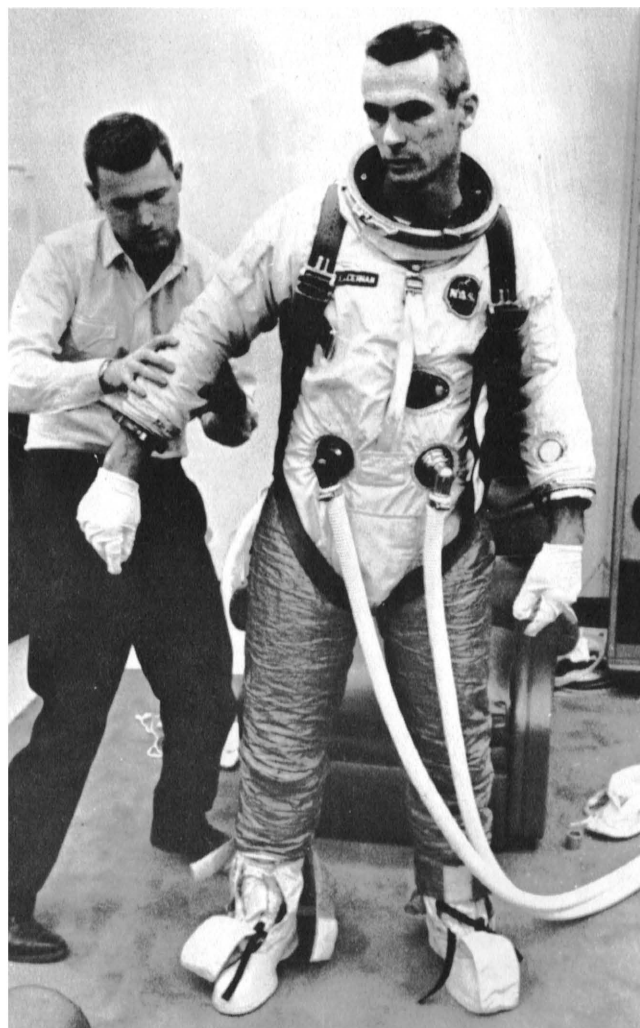
ASTRONAUT EUGENE A. CERNAN , Gemini IX pilot, has his suit adjusted by suit technician Al Rochford in preparation for a test. The Gemini IX extravehicular suit weighed 35 pounds and the leg cover layer was qualified to withstand surface temperatures of 1200 degrees Fahrenheit while maintaining the suit internal temperature to no more than 110 degrees Fahrenheit.
