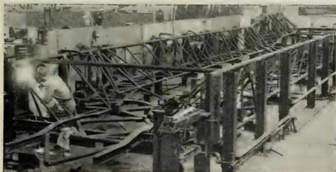
**CRADLE FOR *Atlas* missile begins to take shape as I beams and cross braces are welded together.**
